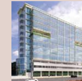
CRESCENT BUSINESS SQUARE
